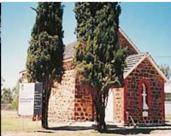
Mingenew church building
